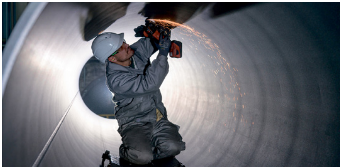
Construction of the pipes for the Nord Stream 2 pipeline.
