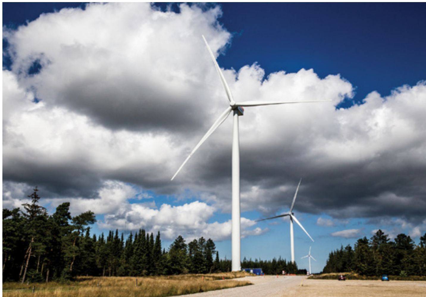
Wind turbines at the National Test Centre for Large Wind Turbines at Østerild, north Jutland. Government investment has supported Denmark's wind energy industry.
