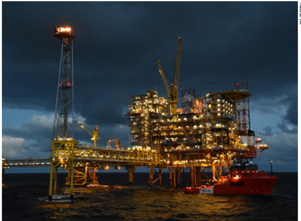
A rig at the Tyra East field in the North Sea. The sinking sea bed is dragging the rigs down with them, making them more vulnerable.
