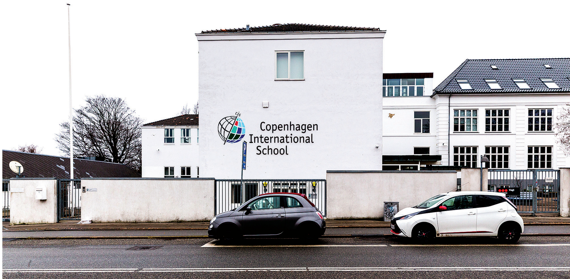
Copenhagen International School's old facilities in Hellerup will soon house around 60 refugees.
