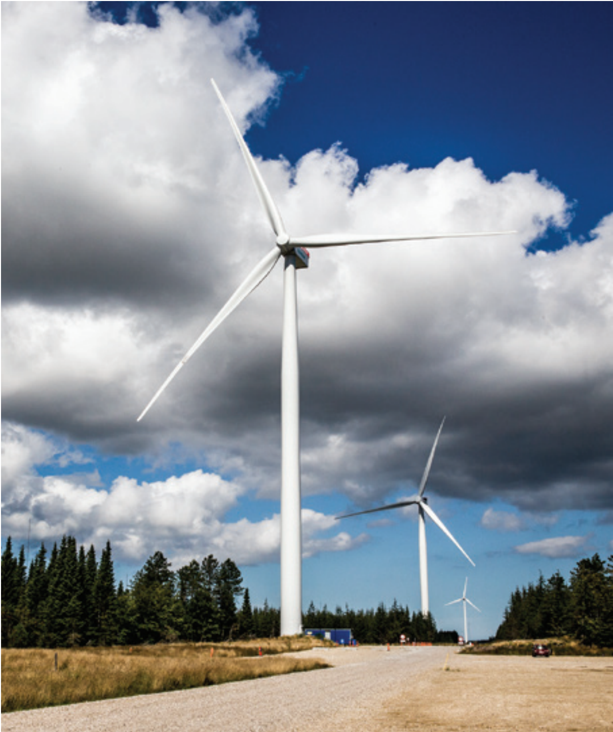
Right: Wind turbines at the National Test Centre for Large Wind Turbines at Østerild, North Jutland. The turbine towers are over 100 metres tall, and the blades more than 70 metres in length. The test centre's geographical location and facilities allow the wind turbine industry, in collaboration with DTU and other research institutions, to carry out research, development and tests of prototype wind turbines and new wind turbine technology.
