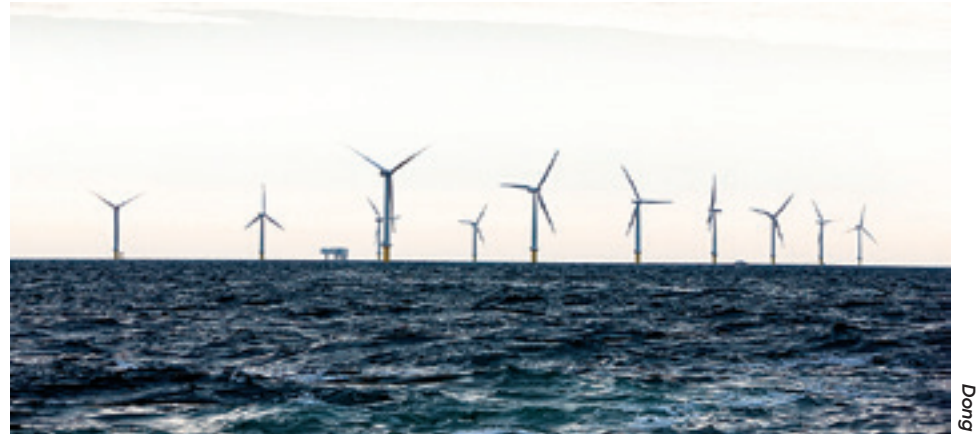
Offshore windmills in the Hons Rev 2 installation.
