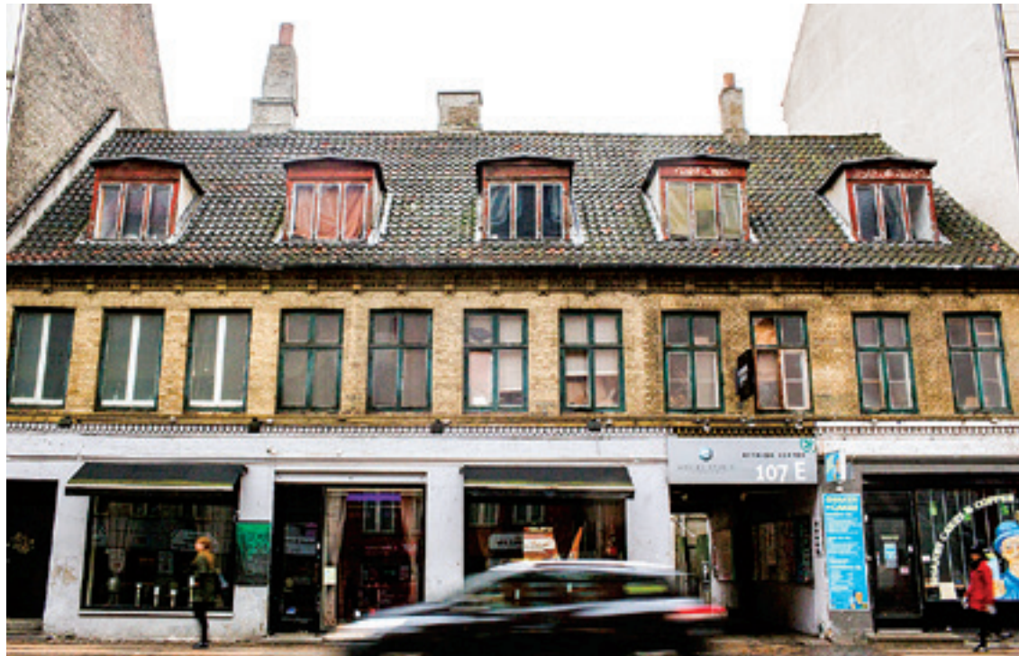
Vesterbrogade 107c, one of the remaining historic buildings on the street, which now faces demolition.
