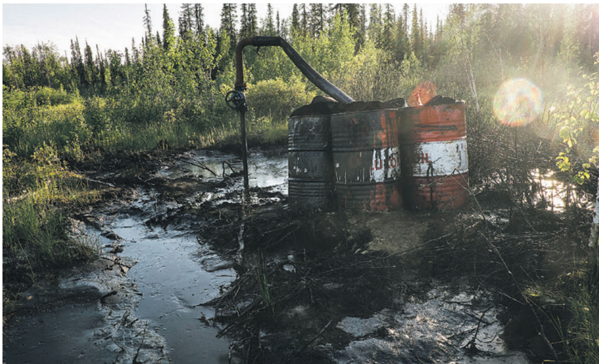
A poorly closed oil well creates a spill in the middle of the Komi forest. Despite being a UNESCO World Heritage Site, oil companies operate with impunity and are unafraid of leaving branded materials as evidence.
