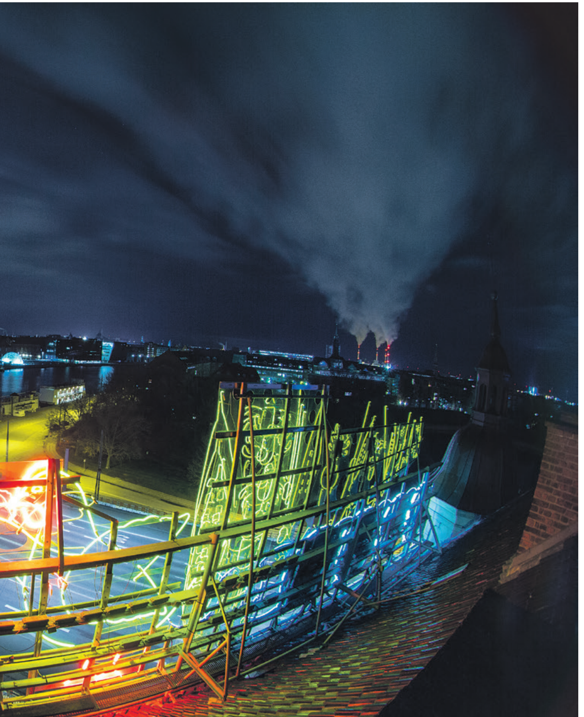
A rooftop view of Copenhagen looking north over the Langebro Bridge. To the east, the Amagerværket power plant releases plumes of white smoke.
